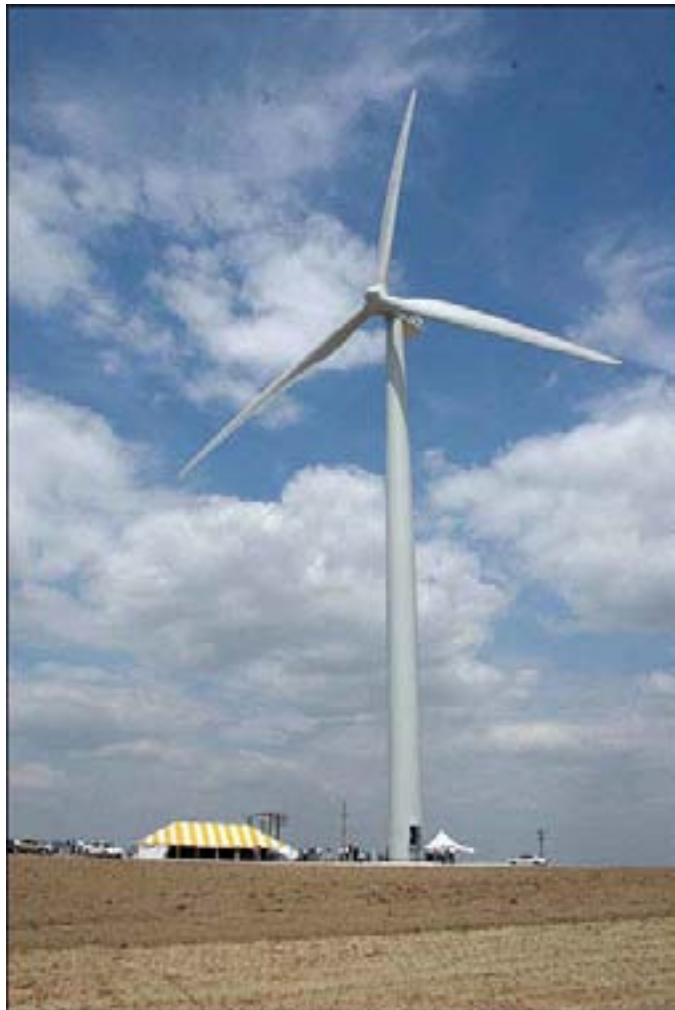
Illinois Rural Electric Cooperative's first wind turbine, completed in May 2005.
